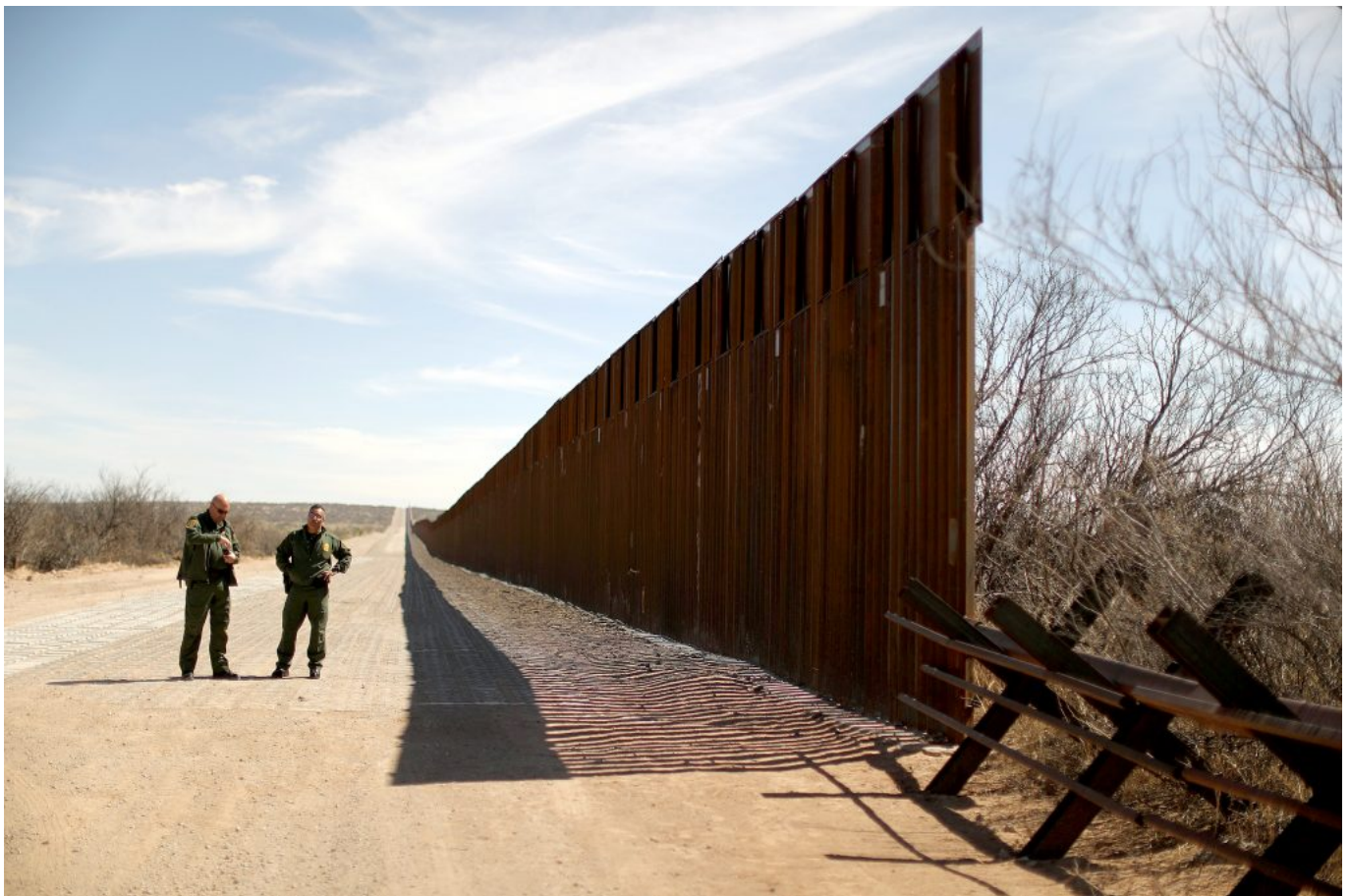
New bollard-style U.S.-Mexico border fencing is seen next to vehicle barriers in Santa
